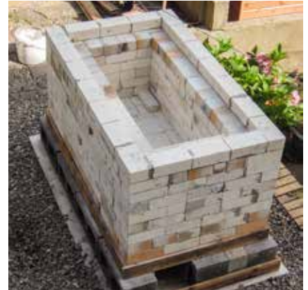
The last brick laid
