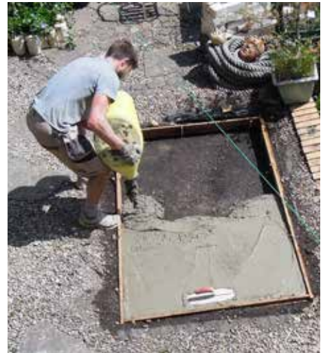
Kiln place and concrete base
