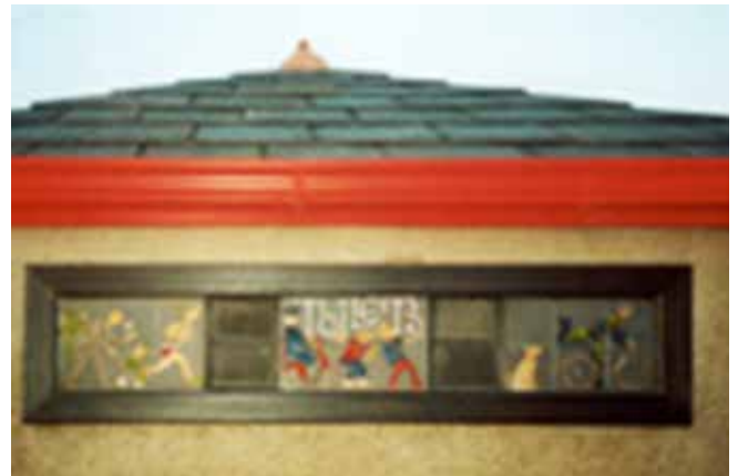
Carnforth public toilets
