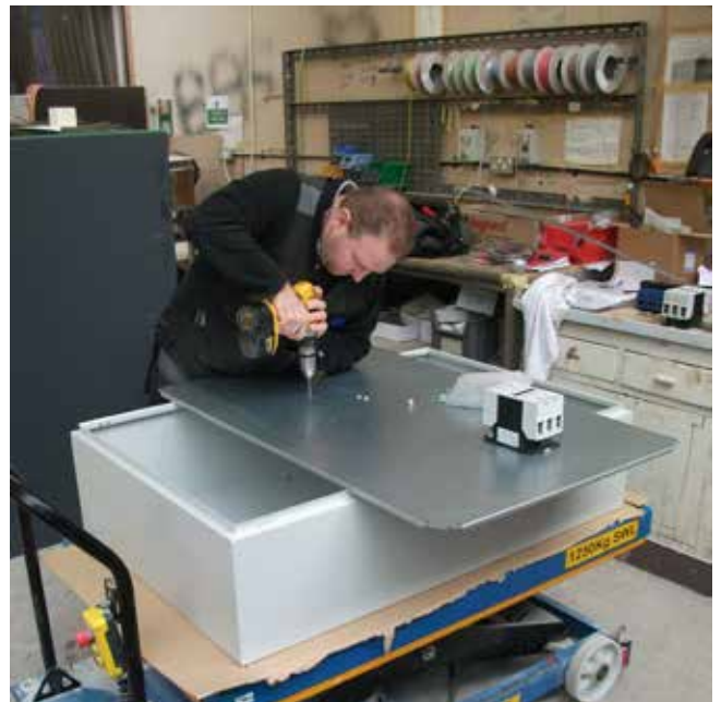
Electrical work on a big kiln
